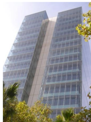
Figure 1– Photography of the building H.
